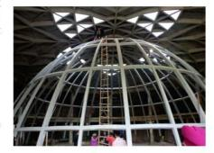
structure. The benefits considered for the design of dome is the ability to cover the large distance with minimum thickness. Structural steel hollow tube sections have been used for the construction of dome
